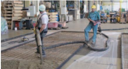
When pumping concrete through hoses, the concrete placement location is often a long way from the pump. With the remote control unit with display, the driver can operate the pump from the placement location and monitor its state.
