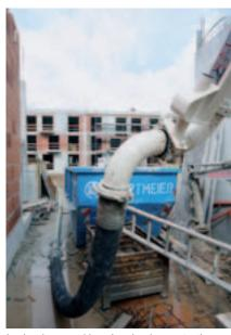
In closely-spaced housing developments, the M 20-4 Sanima is a step ahead: With an extension line connected to one of the boom ends, concrete can be placed over distances that even the long 60 m booms can not span.
