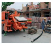
The M 20-4 Sanima as pure hose pump: With the hinged elbow rotated by 180°, reduction couplings for DN 65 delivery hoses can be connected. Here, the M 20-4 Sanima is used in restricted space to pump concrete into cellars through more than 80 m of delivery line.
