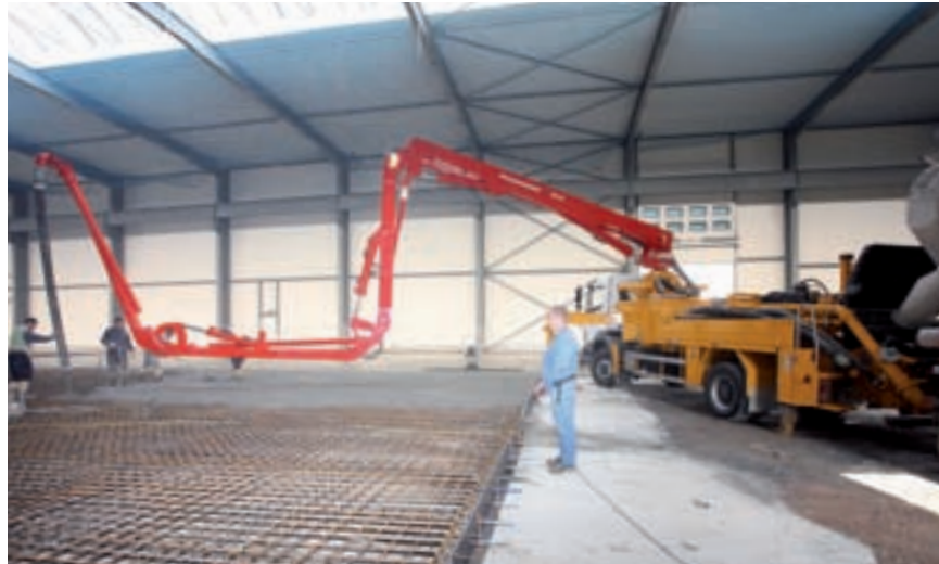
Superior performance when concreting in low buildings – thanks to low unfolding height and flexible roll Z-fold system
