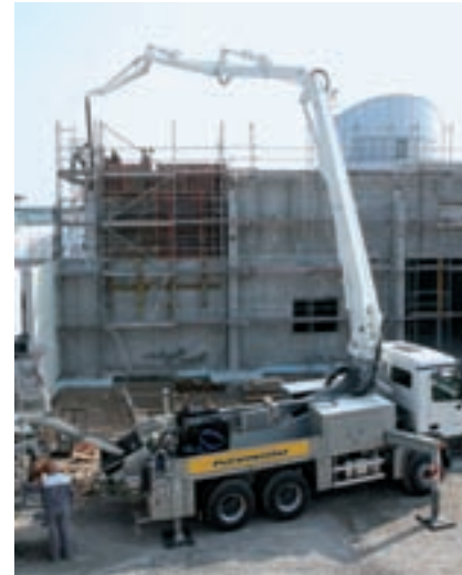
The allrounder on smaller-scale construction sites
