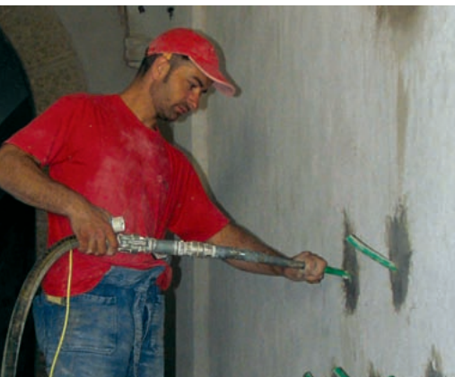
The Sprayboy injecting mortar into the holes.
