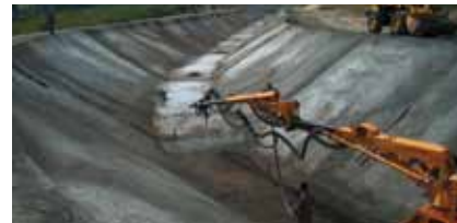
Slope stabilization
