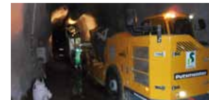
Concrete transport and mixing
